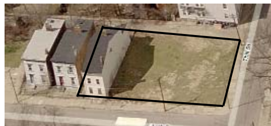
Aerial View of the Site before construction
